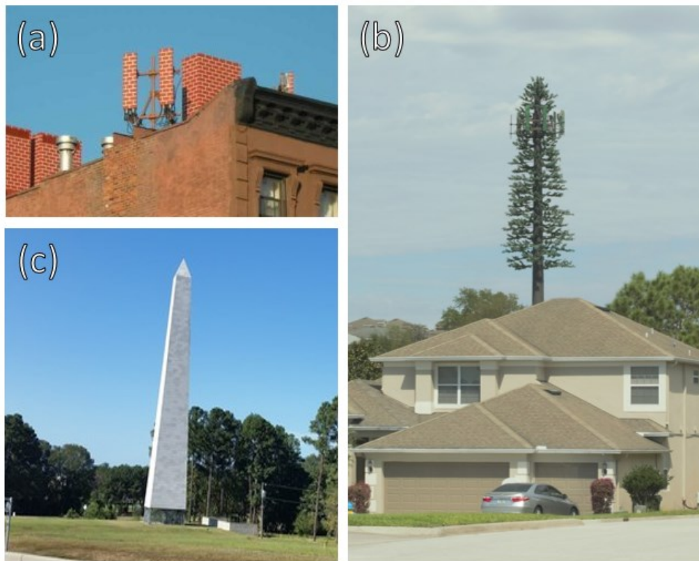
Figure 1 Cellular network base stations disguised to either blend in with the environment or meet city ordinances (a) Cellular network antenna with brick camouflaging pattern [10], (b) Cellular network antenna disguised to look like a tree, (c) Cellular network antenna covered with brick patterned material to look like a stone obelisk to meet city and county ordinances on building exteriors [11].
